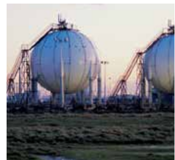
Oil & Gas Transportation & Storage
