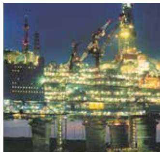
Oil & Gas Processing
